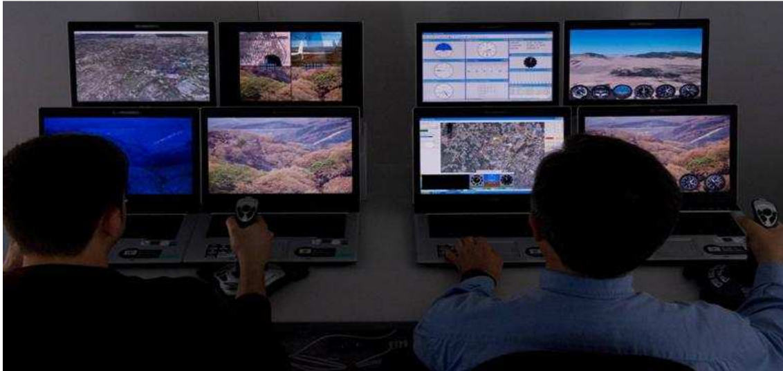
Control station (GCS)
